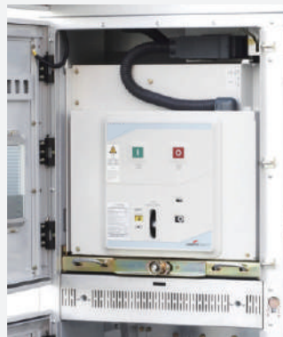
Figure 2/4 Circuit Breaker Compartment
